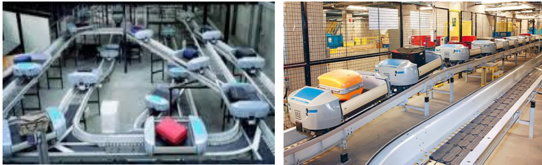
FIGURE 18: DCV baggage handling system (a; b) and late baggage store (c)
