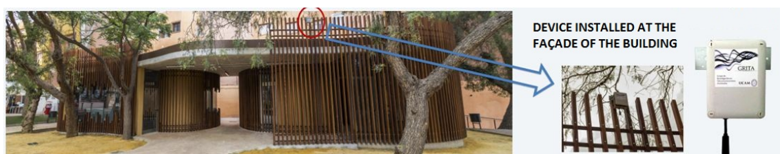
Figure 9. Photography of the multi-purpose room where the devices are installed. A close-up of the outdoor device is shown. Inside of the building there are the gateway, the server and the indoor acoustic device.
