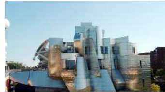
Figura 60: Museo Weisman Vista exterior, Minneapolis, Minnesota 1993, Frank Gehry.
