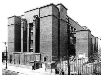
Figura 99: Larkin Building, Buffalo (Nueva York), (1903-1905). Frank Lloyd Wright.
