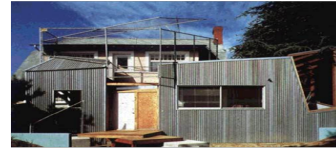
Figura 54: Casa Gehry. Fachada Principal. Santa Monica, 1977 - 1979. Frank Gehry.
